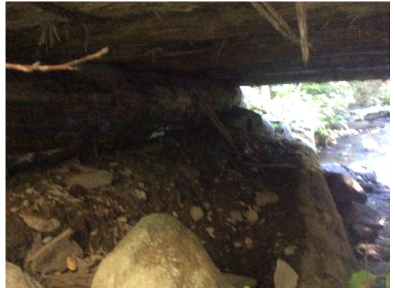
Left Bank Abutment when facing downstream
