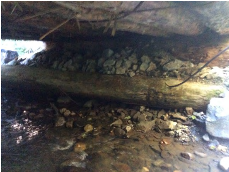
Right Bank Abutment when facing downstream
